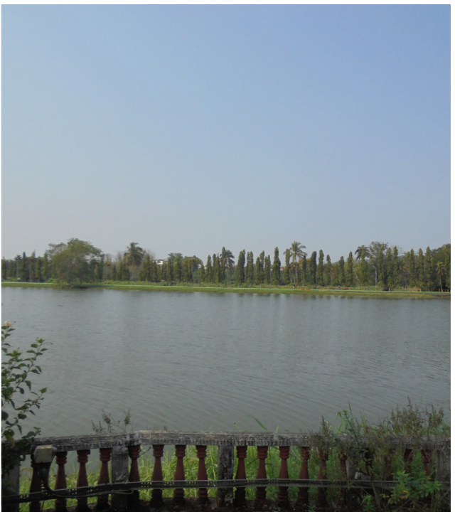
Reservoir -Rainwater Harvesting
