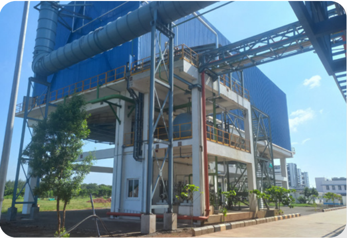
Air Cooled condenser attached with Tuni Co-gen plant
