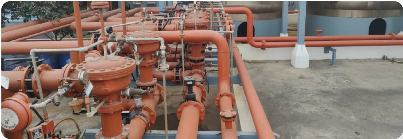
Fire deluge system and Medium Velocity Sprinkler for Bulk storage system
